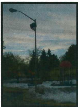
Inadequate outside lighting
